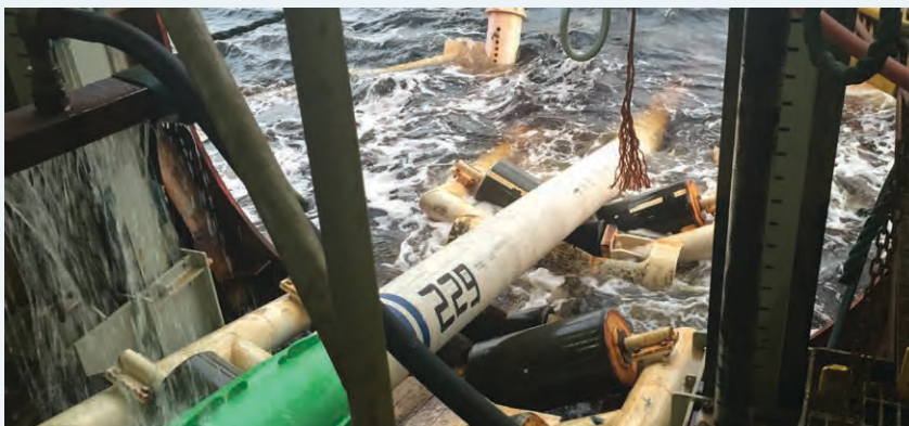
Top left: PIH patented Solaris™ radiant heater. Top right: IMPP station. Bottom: IMPP joint transferring over the stinger
