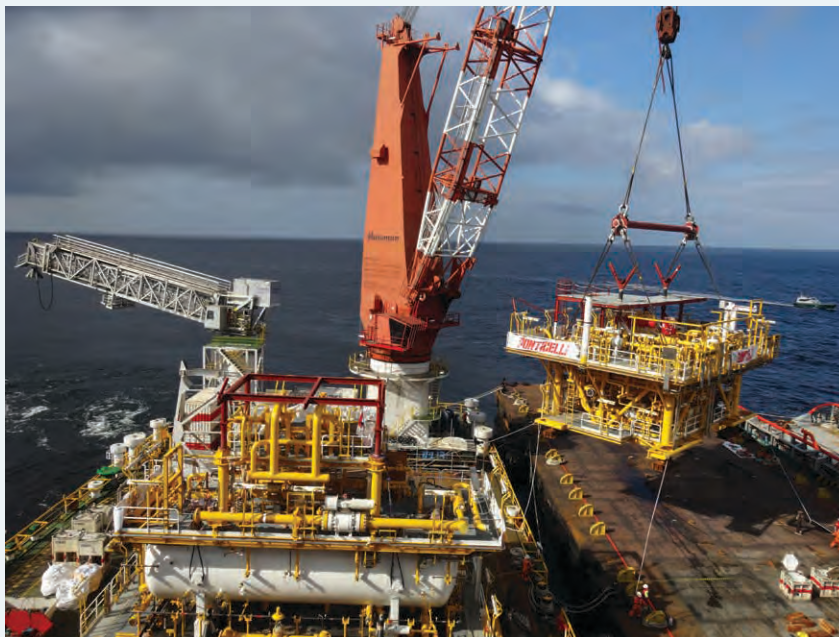
Module installation on Alima FPU.
